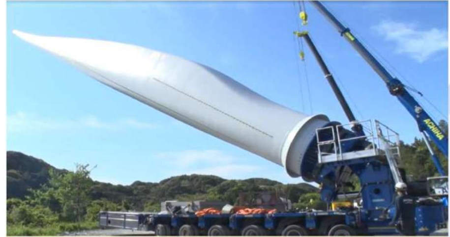
Transportation and Installation
